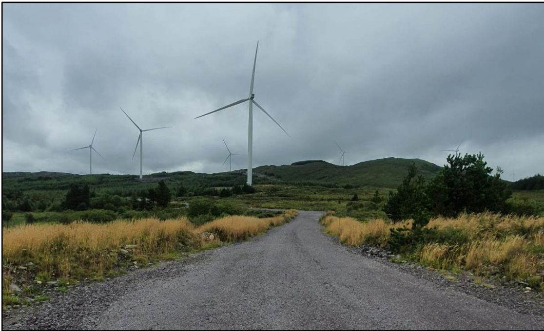
Plate 2.6 Example of reinstated site access track verge with stripped peat material showing signs of revegetation with purple moor-grass ( Molinia caerulea ) and other grass species.
